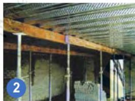
2 Place temporary support if required
