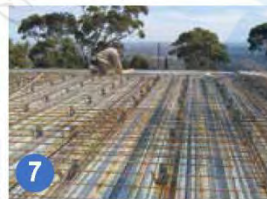
7 Place reinforcement
