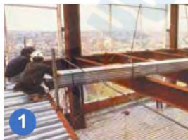
1 Open steel deck sheet bundles
